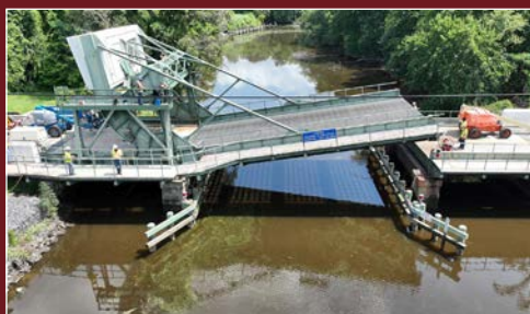
Misphillion Bridge Opens to Traffic
