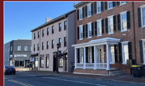
Renovation Completed Downtown
