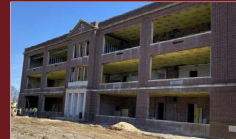
MMS Construction Phase to Begin
